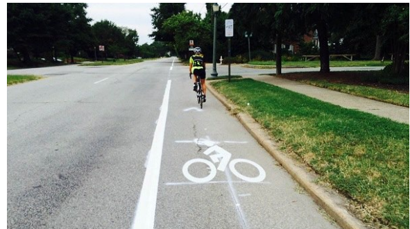
Figure 28. Striped Bicycle Lane on Hermitage Road
