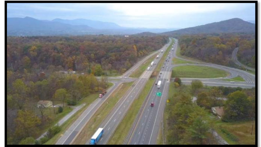
Route 311 (Thompson Memorial Drive)
