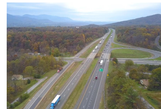
I-81 Exit 140 at Route 311
