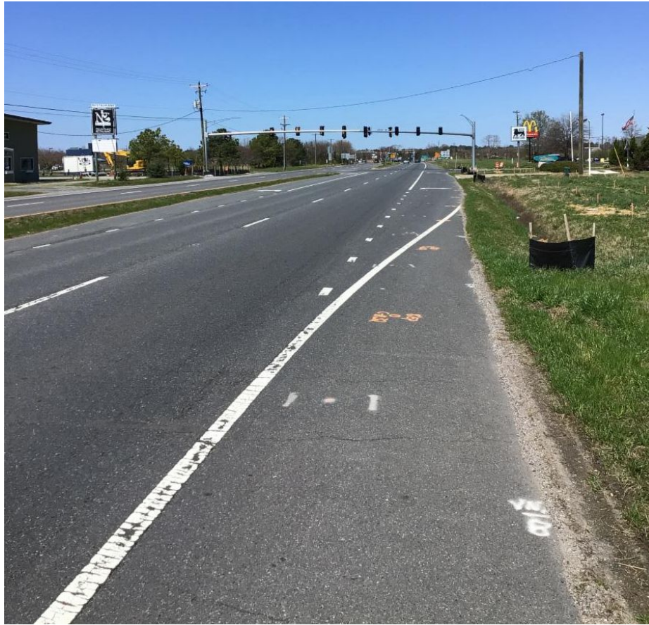
Image: Current view northbound of Route 13 (Lankford Highway) at the entrance to the Food Lion shopping center, and site of new signalized intersection constructed as part of the Route 13 Improvements at Stone Road project. (Traffic signal not operational at this time.)
