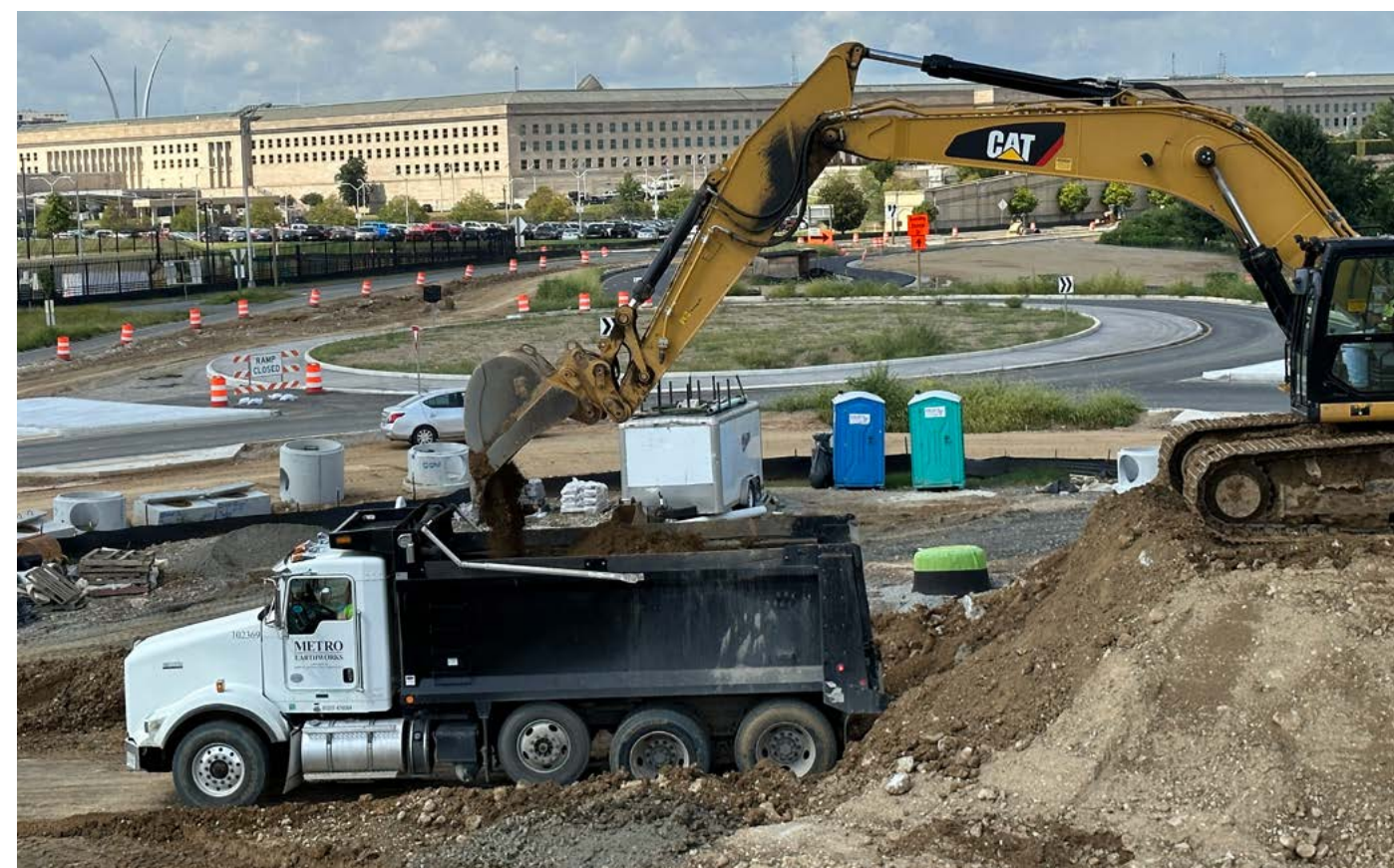
Above: Under Construction — Boundary Channel Drive at I-395 Interchange Improvements
