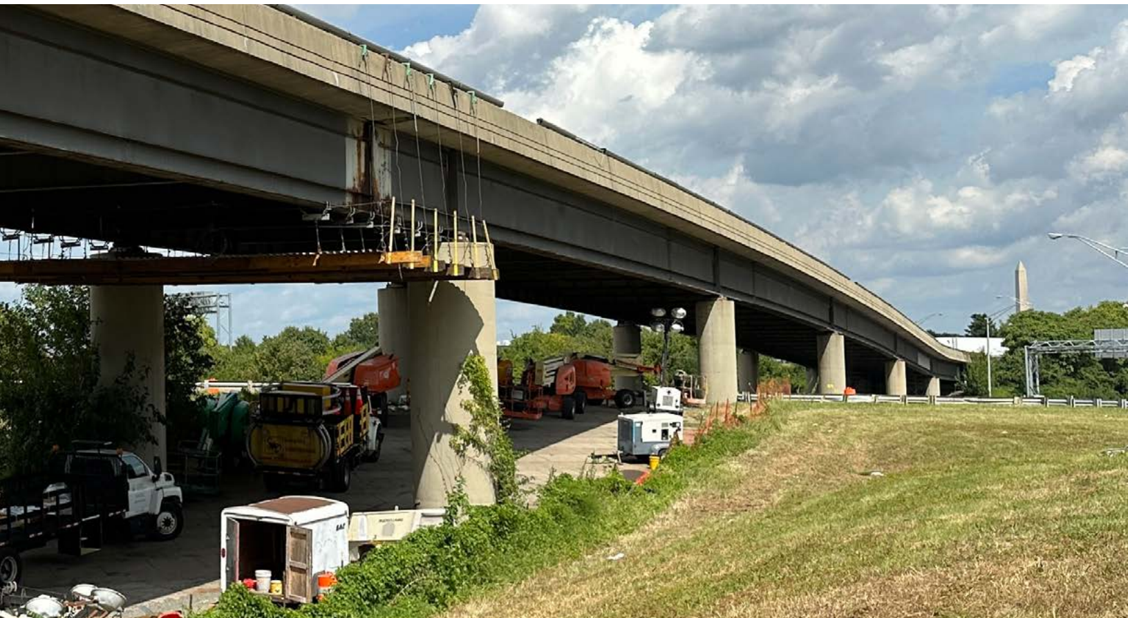
Below: Under Construction — I-395/Route 1 Southbound Exit 8C Bridge Repairs
