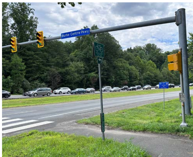
From top: In Design — Fairfax County Parkway Widening at Burke Center Parkway.
