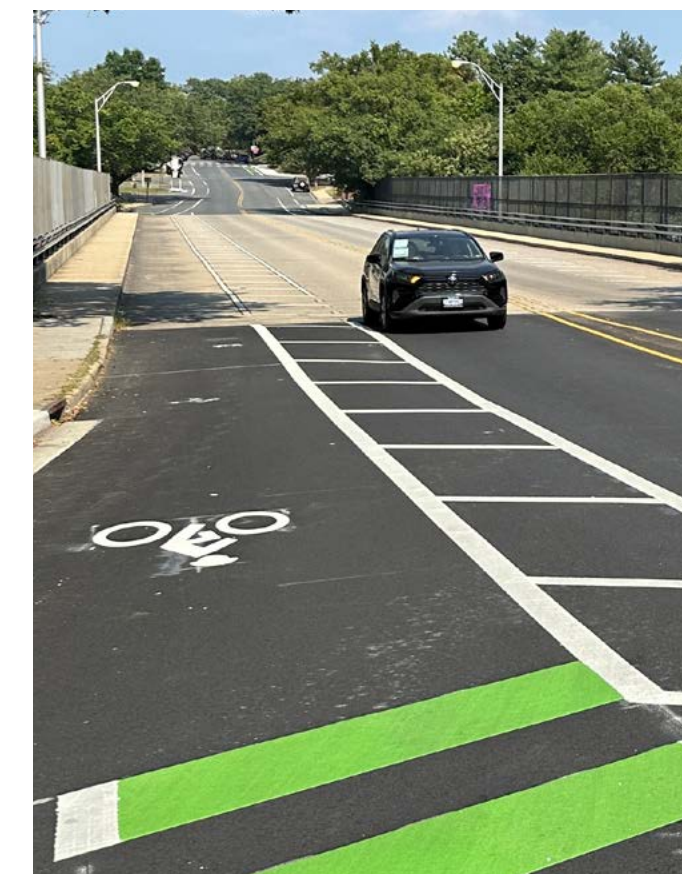
Above: Under Construction — South Abingdon Street over I-395 Bridge Rehabilitation
