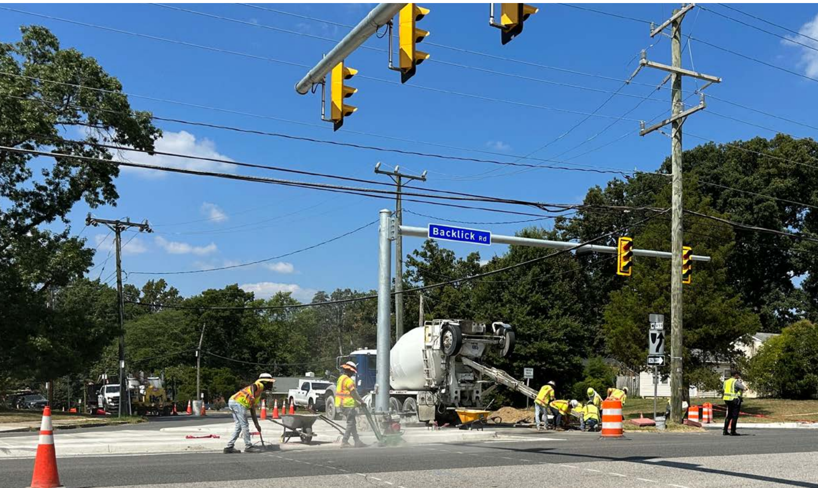
Below: Under Construction — Backlick Road and Leesville Boulevard Intersection Improvements
