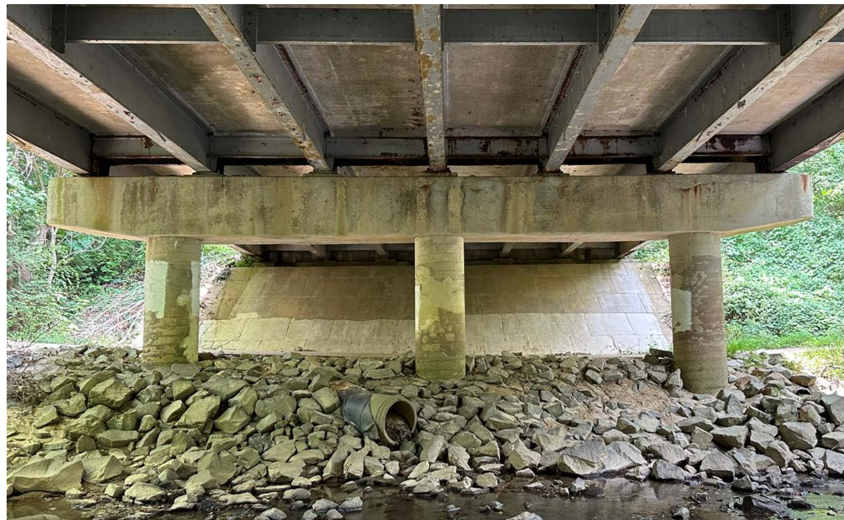
Below: In Design — King Arthur Road over Accotink Creek Bridge Rehabilitation
