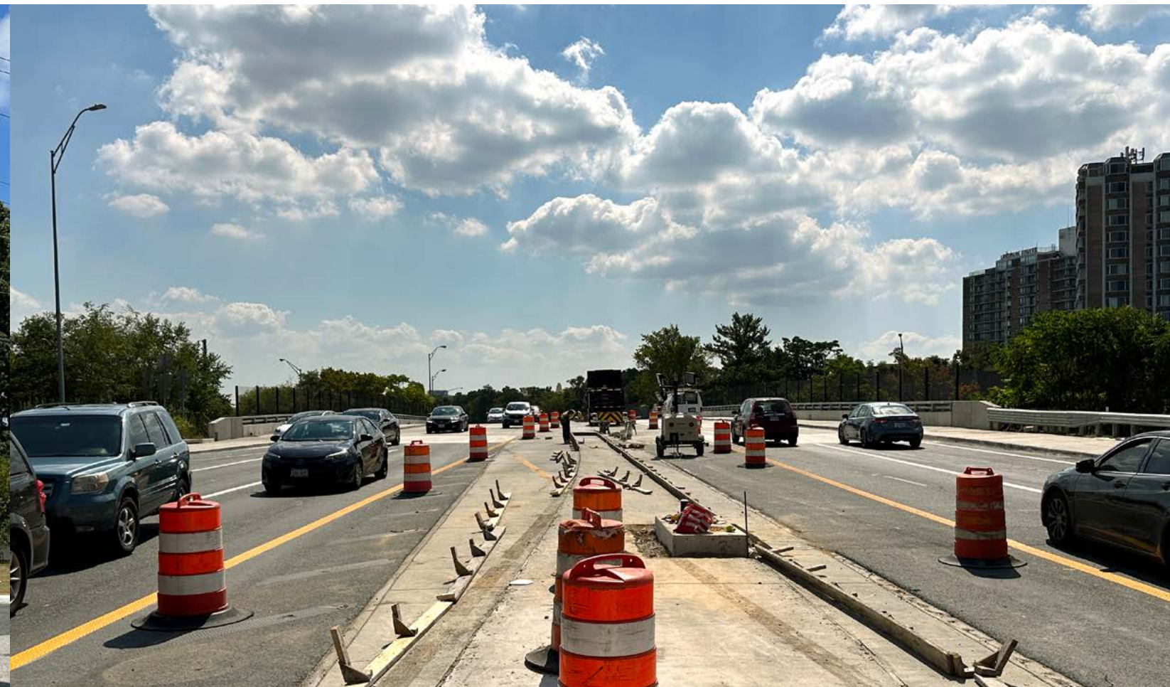
Below: Under Construction — Duke Street over I-395 Bridge Rehabilitation.
