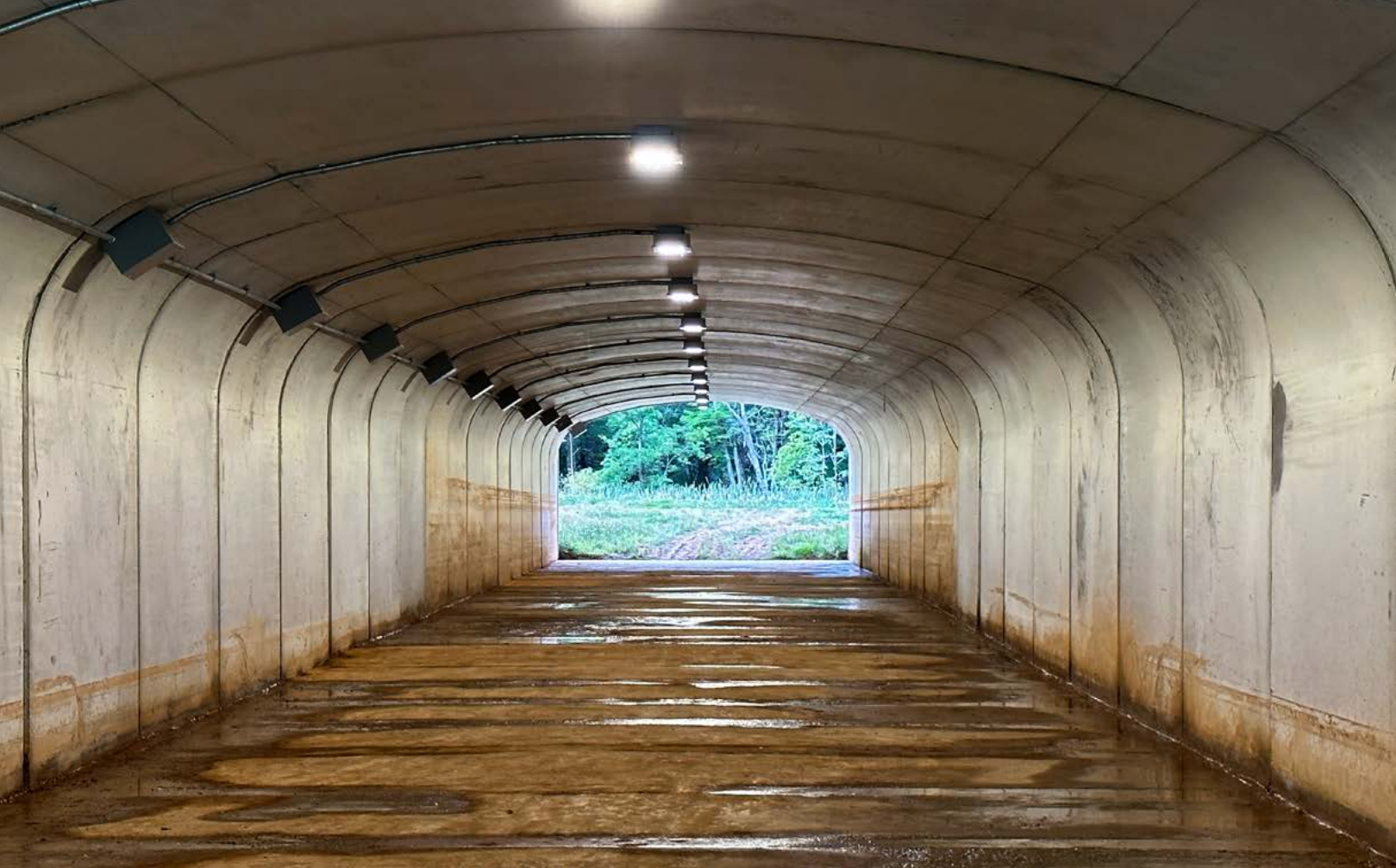
Above: Under Construction— Route 7 Corridor Improvements. Pedestrian underpass.
