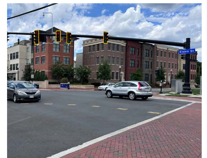
From top: Projects In Design — Braddock Road Multimodal Improvements; Compton Road Shared-Use Path; Elden Street Widening and Underground Utilities Duct Bank
