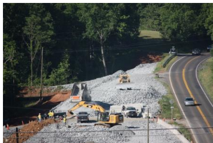
Figure 3. Route 340 Bridge Replacement
