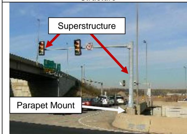
**Figure 9 – Parapet Mount - Traffic Signal Structure**
