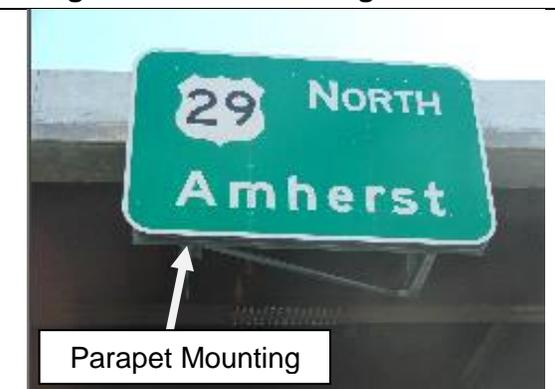
**Figure 4 – Parapet Mount Sign Structure**
