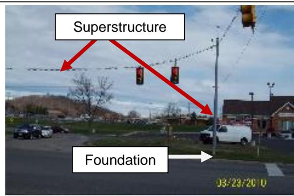
**Figure 8– Span Wire Traffic Signal Structure**
