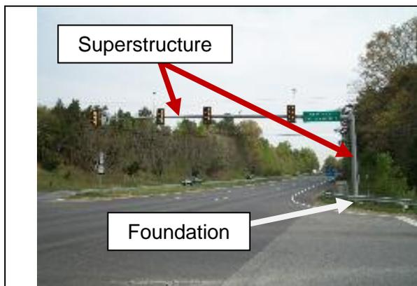
**Figure 7 – Cantilevered Arm Traffic Signal Structure**
