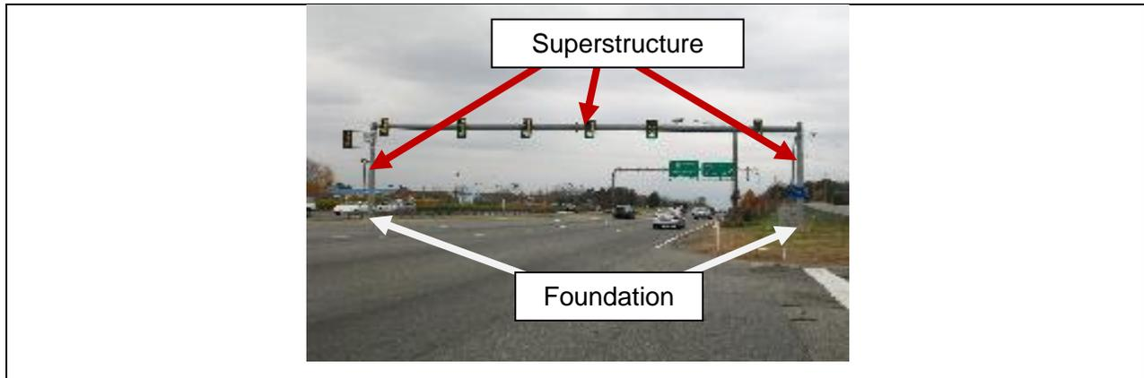
**Figure 11 – Overhead Traffic Signal Structure**
