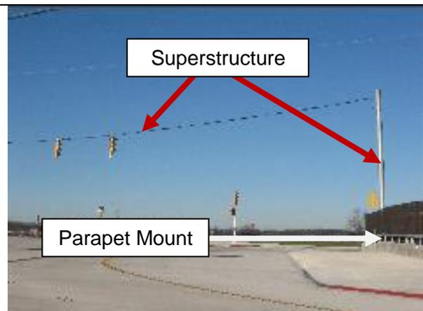
**Figure 10 – Parapet Mount - Traffic Signal Structure**
