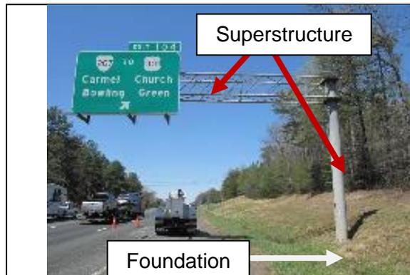
**Figure 1 – Cantilever Sign Structure**
