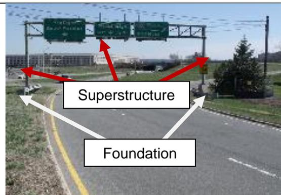
**Figure 2 – Overhead Sign Structure**
