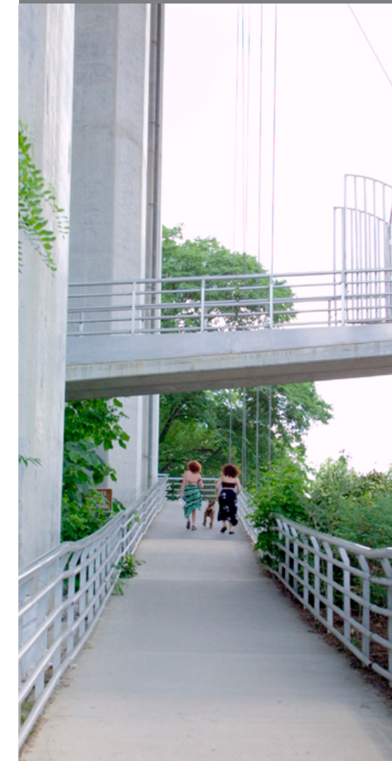
Location: Belle Isle Footbridge, Richmond VA
