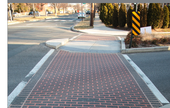
Stamped asphalt crosswalk. Location: N Brookside Drive and Washington Blvd., Arlington, VA
