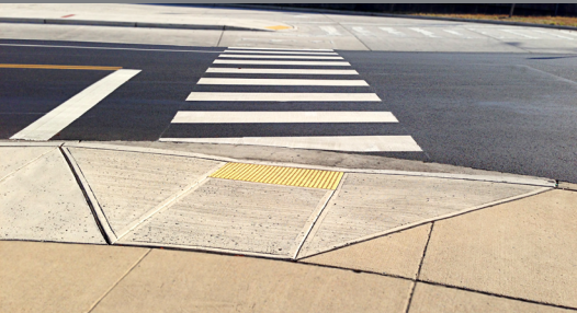
Typical ADA curb ramp, high-visibility crosswalk, and vehicle stop bar. Location: S Quincy St., Arlington, VA
