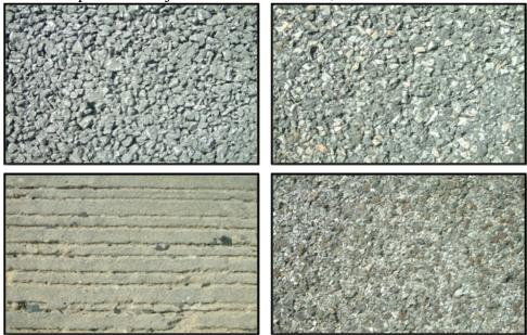
Figure 32. Smart Road surfaces measured. Clockwise from top left: Quiet pavement, inbetween, standard asphalt, and concrete.
