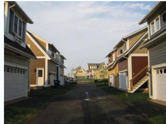
Alleys allow parking, trash collection, and other service functions to be neatly organized out of sight.
